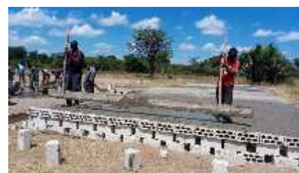
At the time of our visit we had just finished the Foundation Slab.
